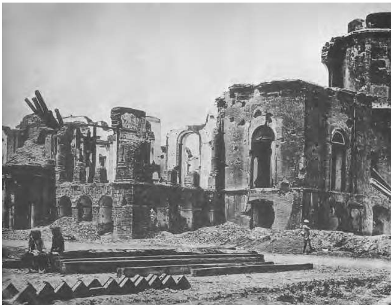
Fig. 12 – Ruins of the Residency in Lucknow
