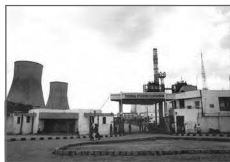
Fig 3.12: A view of a Thermal Power Station
