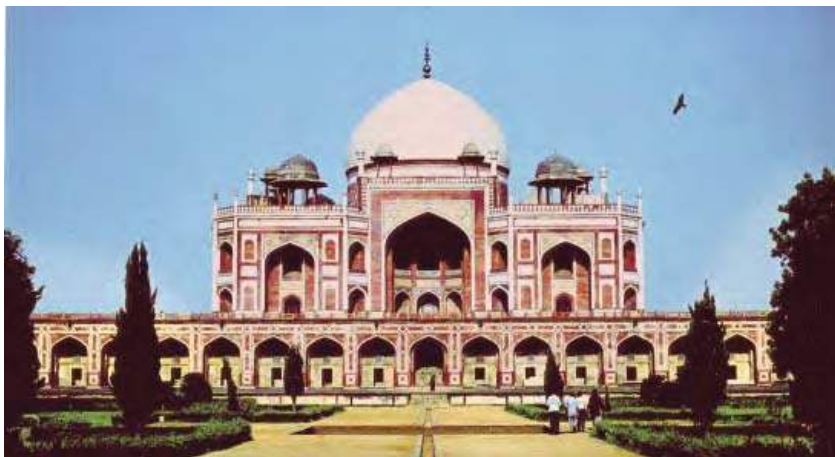
Fig. 11 Tomb of Humayun, constructed between 1562 and 1571. Can you see the water channels?
