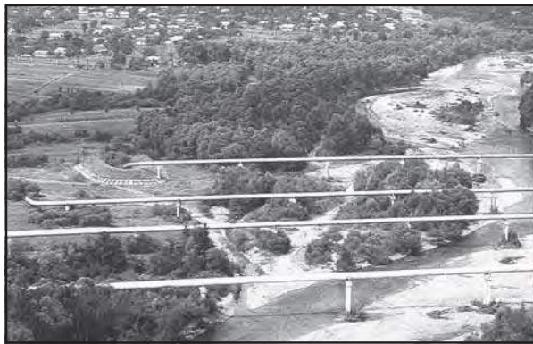
Fig. 8.17: Pipelines transporting natural gas in Ukraine
