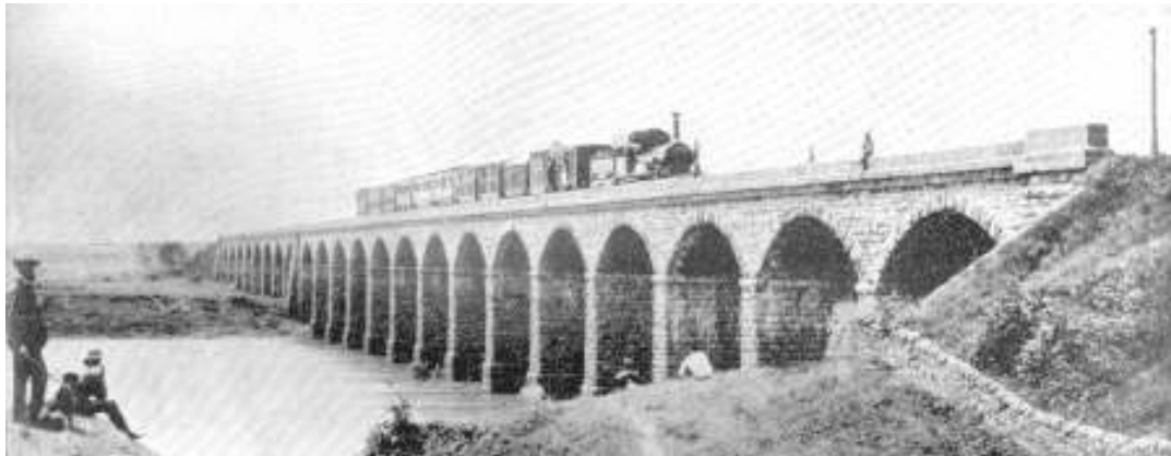
Fig. 1.4 First Railway Bridge linking Bombay with Thane, 1854
