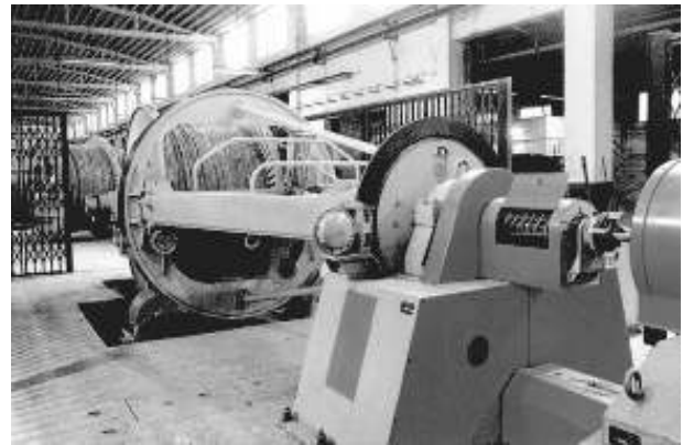
Fig. 6.9: Cable manufacturing facilities at HCL, Rupnarainpur (West Bengal)
